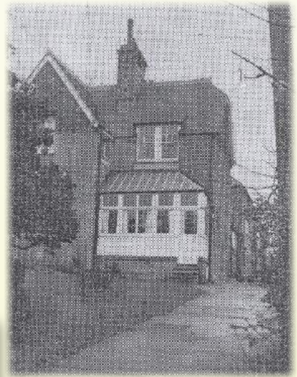
Above: The Gables, an old house that was converted into flats during the 50's was demolished to make way for the new Park Lane Church
